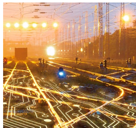
Modern railway infrastructure with surge protection
